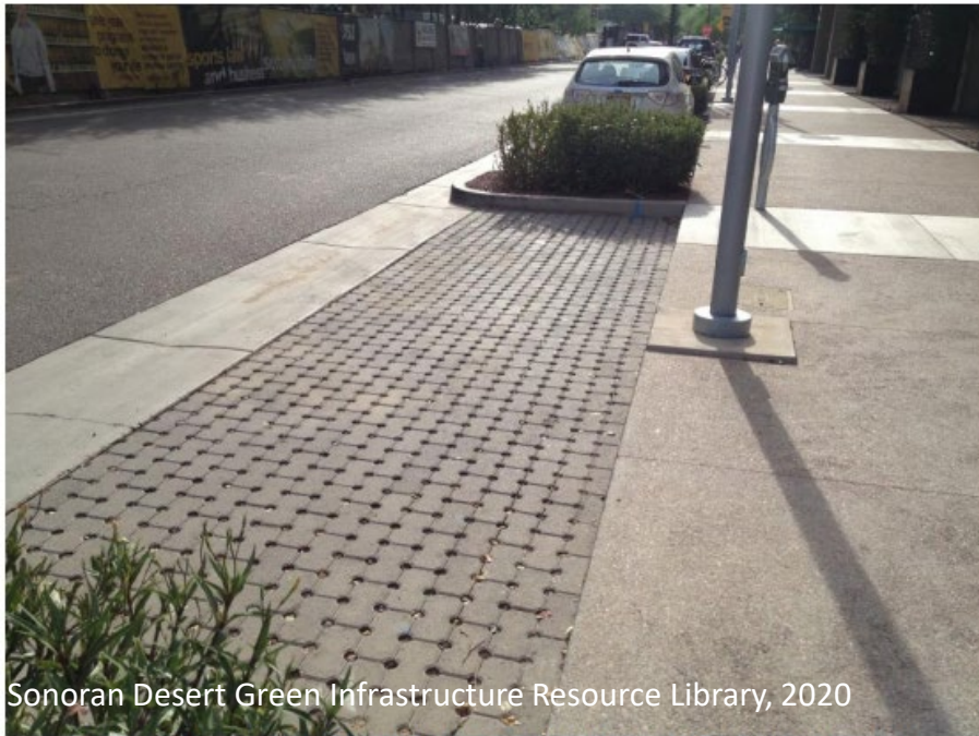
Figure 7: Pervious Pavers (Interlocking Porous Concrete Pavers) Source: City of Phoenix, Office of Environmental Programs.
