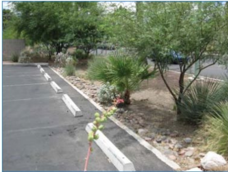
Bioretention basins, like this one between a restaurant parking lot and the street, capture and filter stormwater. Landscape area is graded below the level of the parking lot.
