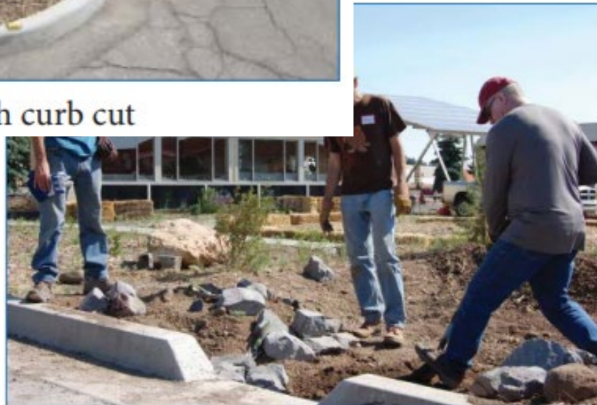
Curb cuts on a street in Flagstaff, AZ (left) and curb cores on a street in Tucson (right) are used to direct stormwater runoff from the street into basins before pollutants reach washes and rivers.
