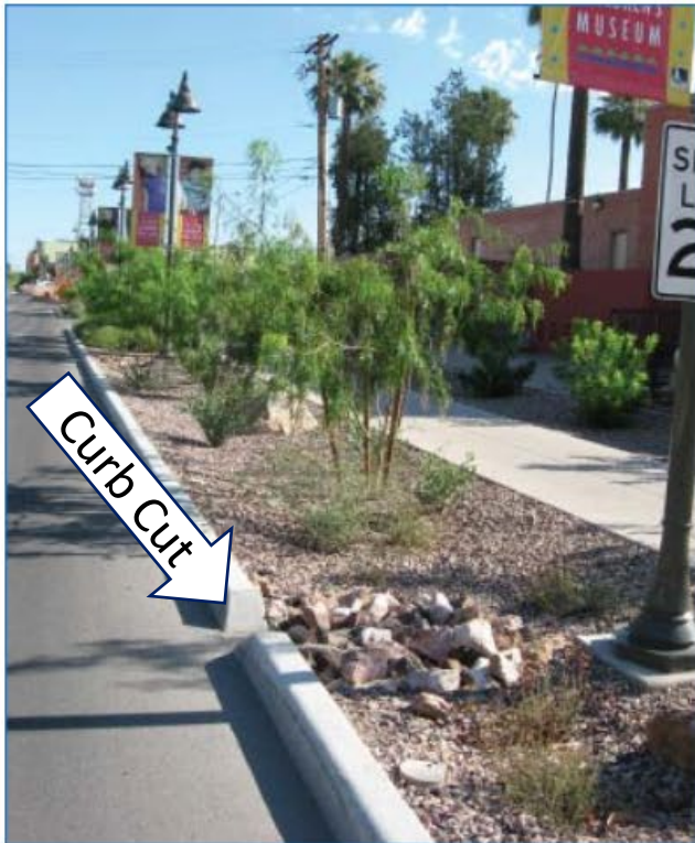
This long, shallow swale in the right of way has multiple curb cuts along its length.
