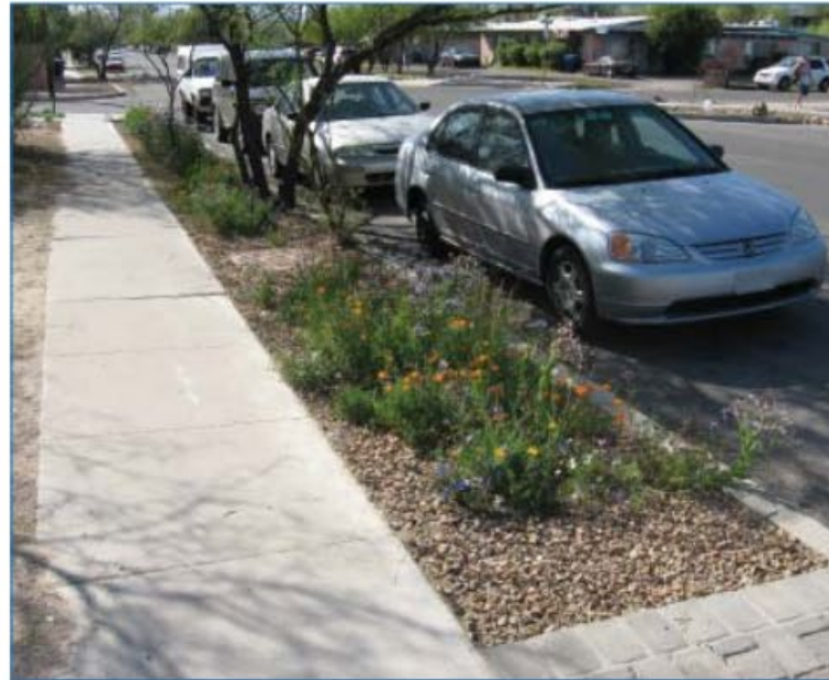
At this site in Tucson, a 3" deep swale was created in the ROW to collect runoff from the sidewalk and adjacent property.
