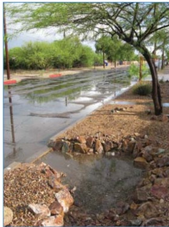
Sedimentation and absorption occur when stormwater is slowed down and is allowed to pool in basins.
