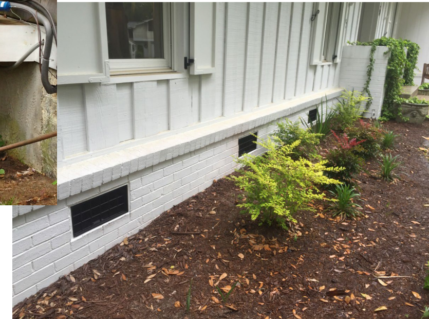
Flood vents allow water to enter the basement, preventing excessive pressure from developing on the basement walls. ( floodflaps.com/new-construction/ )
