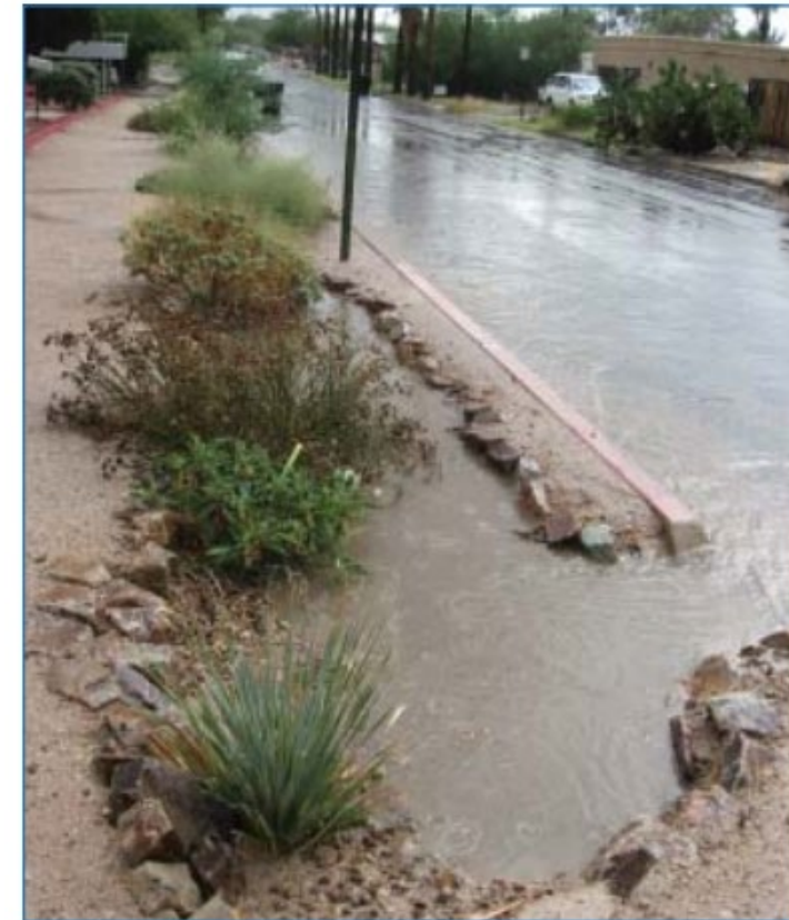
A curb cut draws stormwater from the street into a bioretention basin in the right-of-way.
