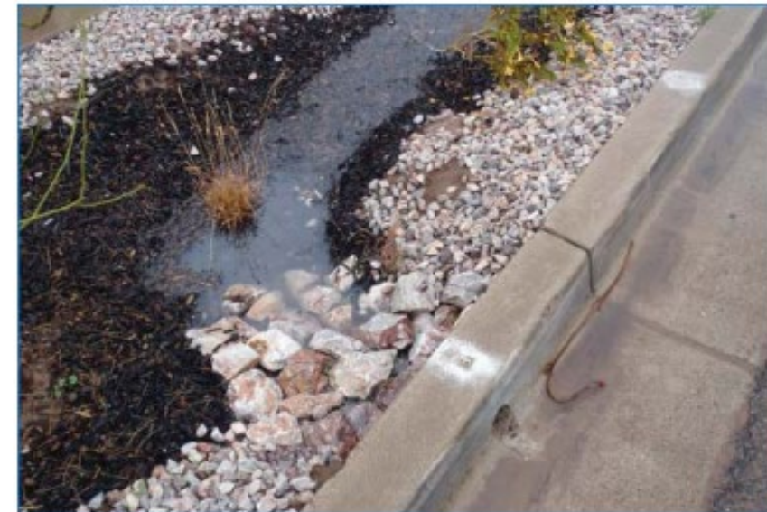
Curb cuts on a street in Flagstaff, AZ (left) and curb cores on a street in Tucson (right) are used to direct stormwater runoff from the street into basins before pollutants reach washes and rivers.
