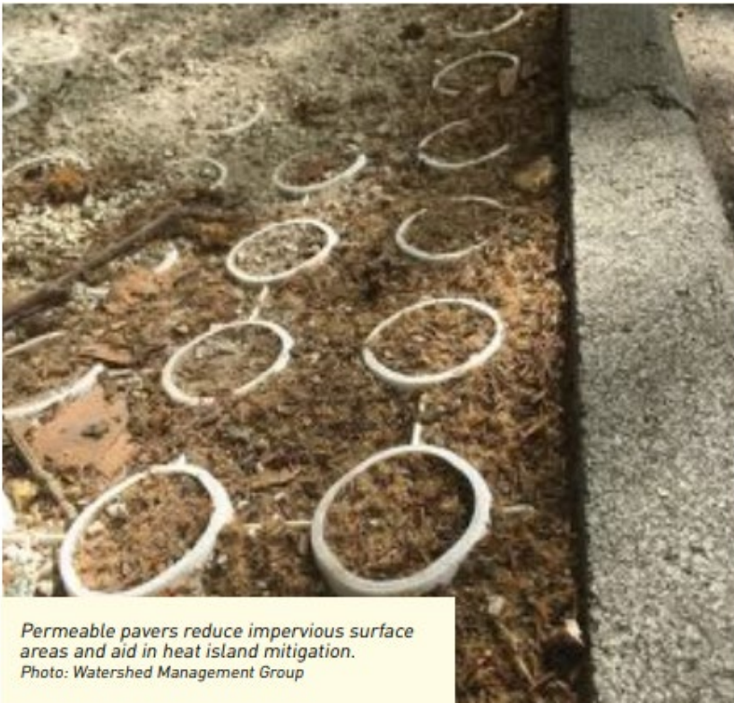
Figure 7: Pervious Pavers (Interlocking Porous Concrete Pavers) Source: City of Phoenix, Office of Environmental Programs.
